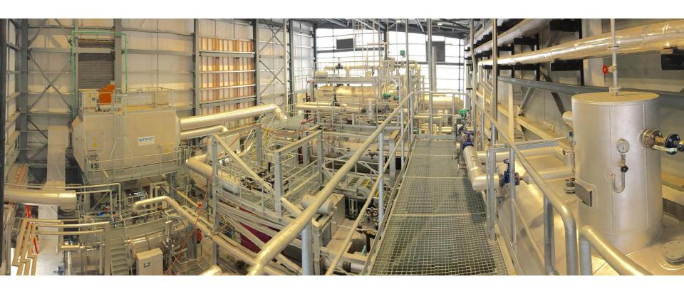
After running 30,000 km of cables, 1,000 m of pressure pipe work, over 2,500 pipe welds with 10% being subjected to radiographic testing without a single failure and the installation of several hundred tonnes of equipment, the commissioning of the plant was, not surprisingly, carried out without any problems!
