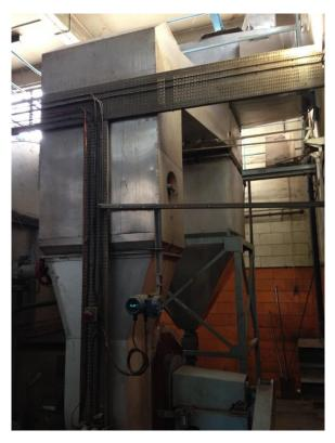
The two 2.85MW coal fired boilers were commissioned in 1964 and are coal fed chain grate fire tube boilers. In Winter they use up to 7 tonnes of coal each day and 3-4 tonnes in Summer.
