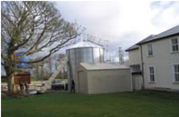
Fuel being conveyed
